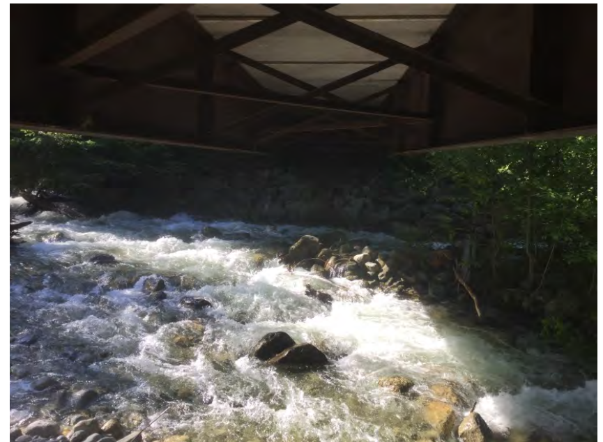
Left Bank Abutment when facing downstream
