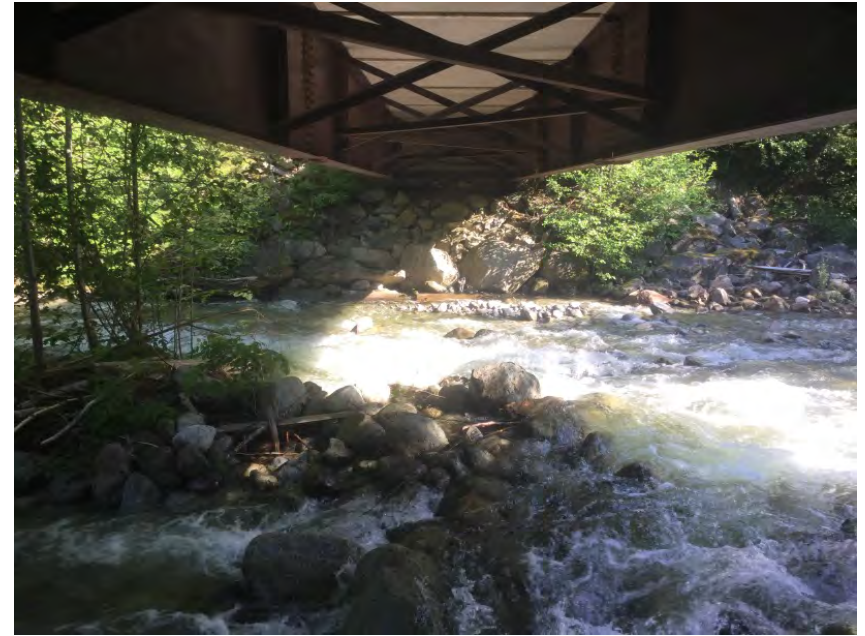
Right Bank Abutment when facing downstream
